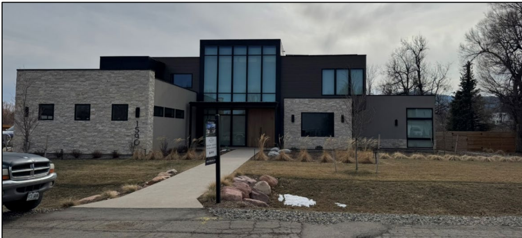
Figure 1: Recently Completed Replacement Home
