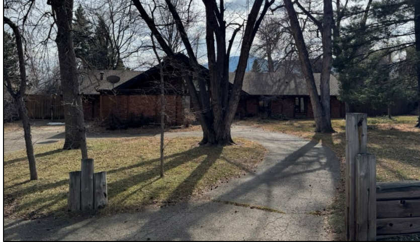
Figure 3: Home Approved for Demolition and Replacement
