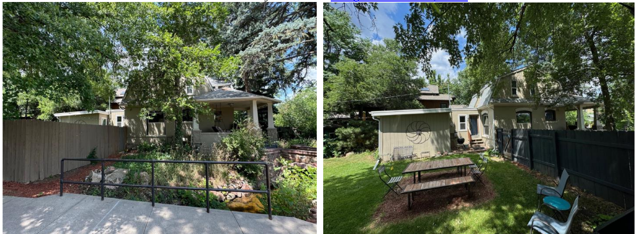
Figure 2. Left: North end of east elevation from 7 th Street showing the east facing part of the gambrel roof and the hipped roof of the existing front porch. Right: South end of east elevation showing the flat roof addition to the south side of the house. Provided by applicant.
