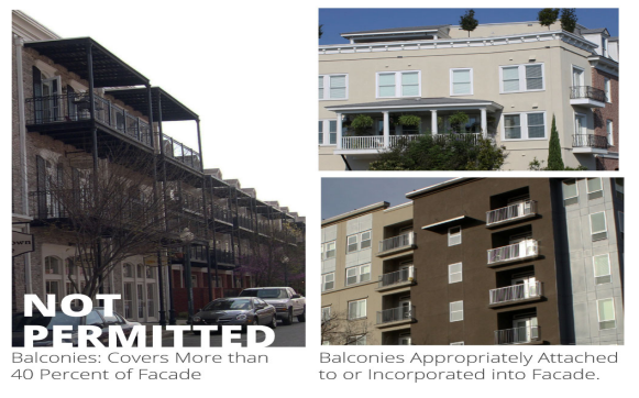
Figure 14-65. Examples of Balconies
