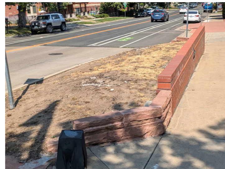
VIEW LOOKING EAST
