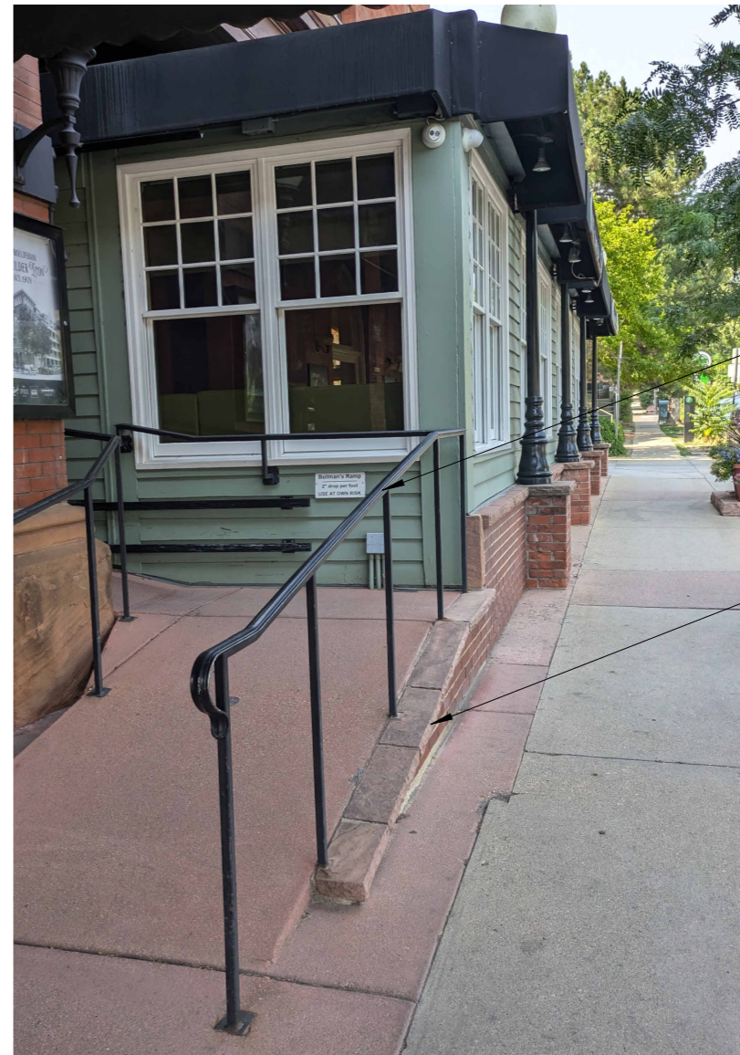
VIEW LOOKING NORTH
