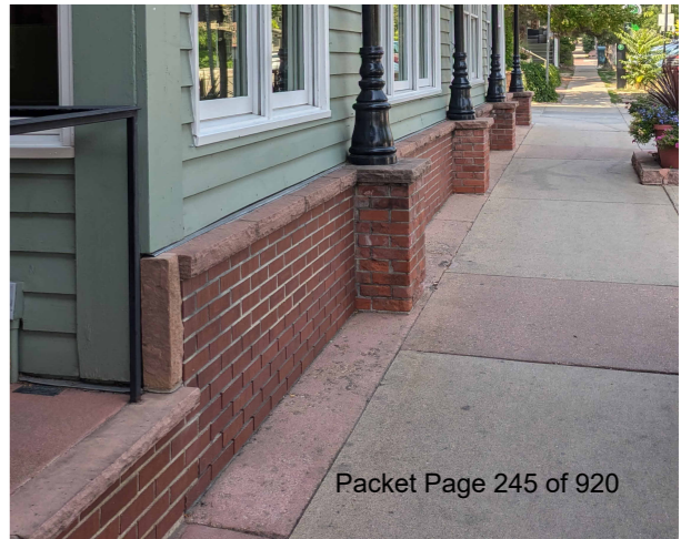
VIEW LOOKING NORTH
