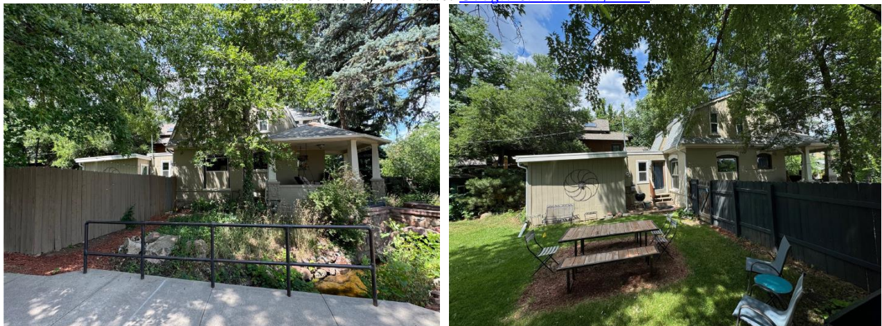
Figure 2. Left: North end of east elevation from 7 th Street showing the east facing part of the gambrel roof and the hipped roof of the existing front porch. Right: South end of east elevation showing the flat roof addition to the south side of the house. Provided by applicant.
