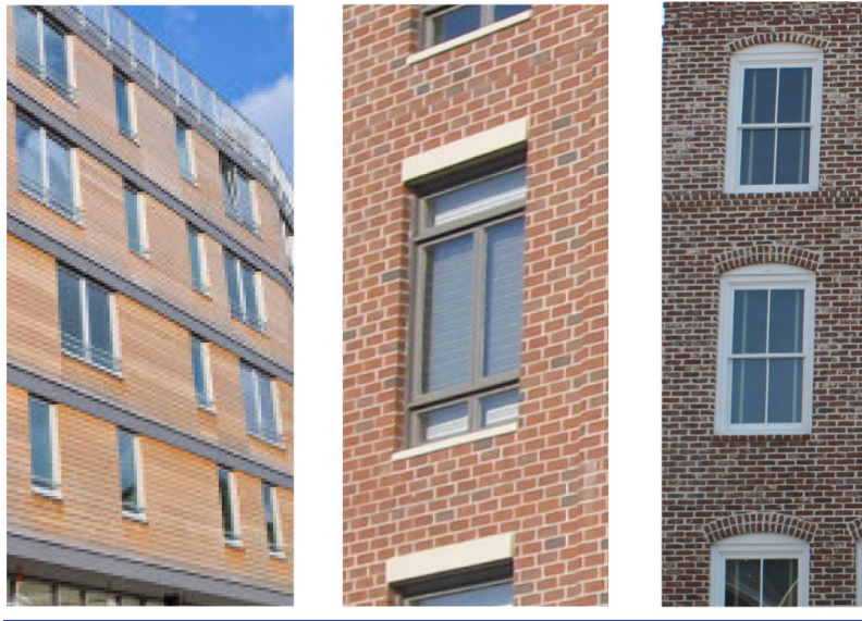
Figure 14-63. Vertically Oriented Windows with Expressed Lintels
