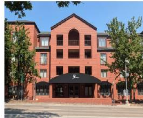
VIEW LOOKING EAST
