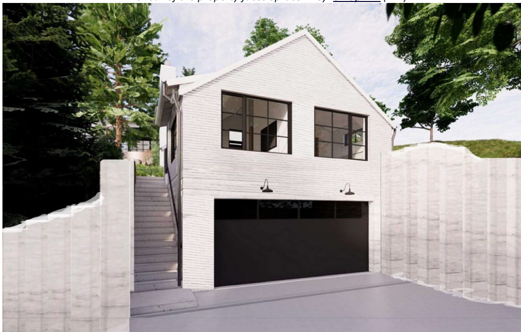
Figure 2. Proposed south elevation (view from alley) of proposed new accessory building showing the 25 feet height of the proposed new building, 8 in 12 pitched roof with dormers, steps up to grade at the west (left) side and flanking limewash engineered concrete walls.
