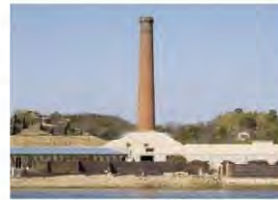
Inujima Seirenscho Art Museum Inujima Island, Japan Designation: National Heritage Site This small isle in the Sea of Japan was occupied by a copper refinery built in 1909. It closed around 1920, and by 2008 only a few remnants remained. These, prominently including the smokestack, were included in a new art museum constructed on the site.
