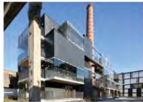
Savonnerie Heymans Brussels, Belgium Designation: No MDW Architecture opted to retain many of the industrial features of this former soap factory complex when converting it into social housing. Pictured above is an apartment block which was built around the plant's smokestack. It is used to ventilate the apartments' underground parking area.
