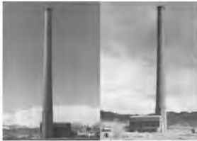
Ohio-Colorado Smelting and Refining Company Smokestack Salida, CO Designation: National Register An imposing, 365' smokestack is one of the few remaining artifacts of the once thriving smelter at Salida, which closed in 1922. It has been placed on the National Register of Historic Places as "a highly visible monument to the industry of mining, an industry vital to the settlement of Colorado."
