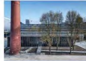
Boiler House Ceres Eindhoven, the Netherlands Designation: No Originally the campus boiler house for Eindhoven Technical University, this facility was heavily renovated into a chemistry lab. One element that was preserved relatively intact was the boiler house's brick smoke stack, standing as a reference to the facility's utilitarian past.
