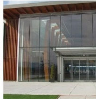
Glass Curtain Wall
