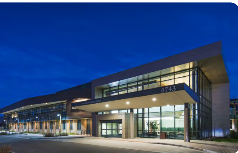
Anderson Medical Center with rooftop solar
