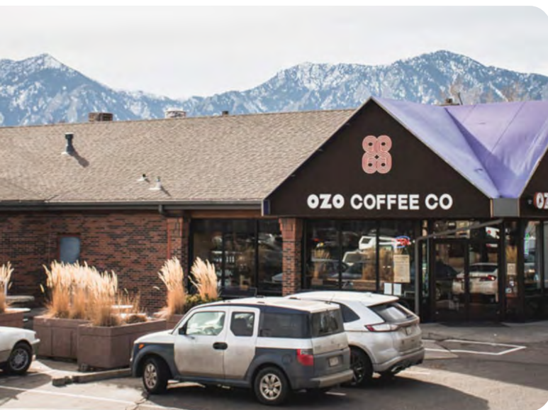
Commercial plaza on the south end of station area
