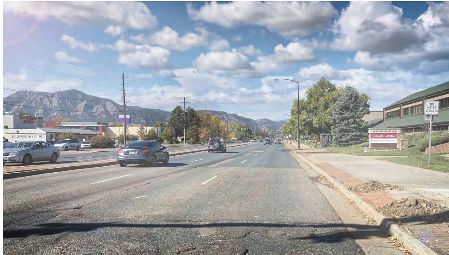
Arapahoe Avenue, Looking West – Existing Condition
