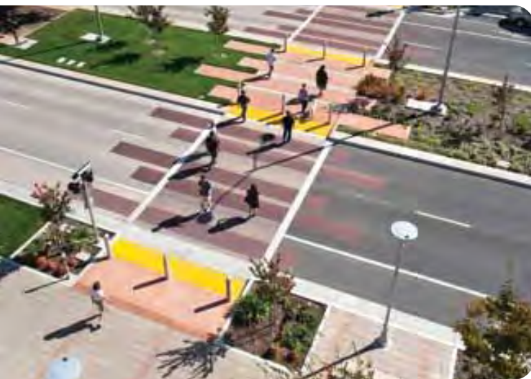
Enhanced midblock pedestrian crossing
