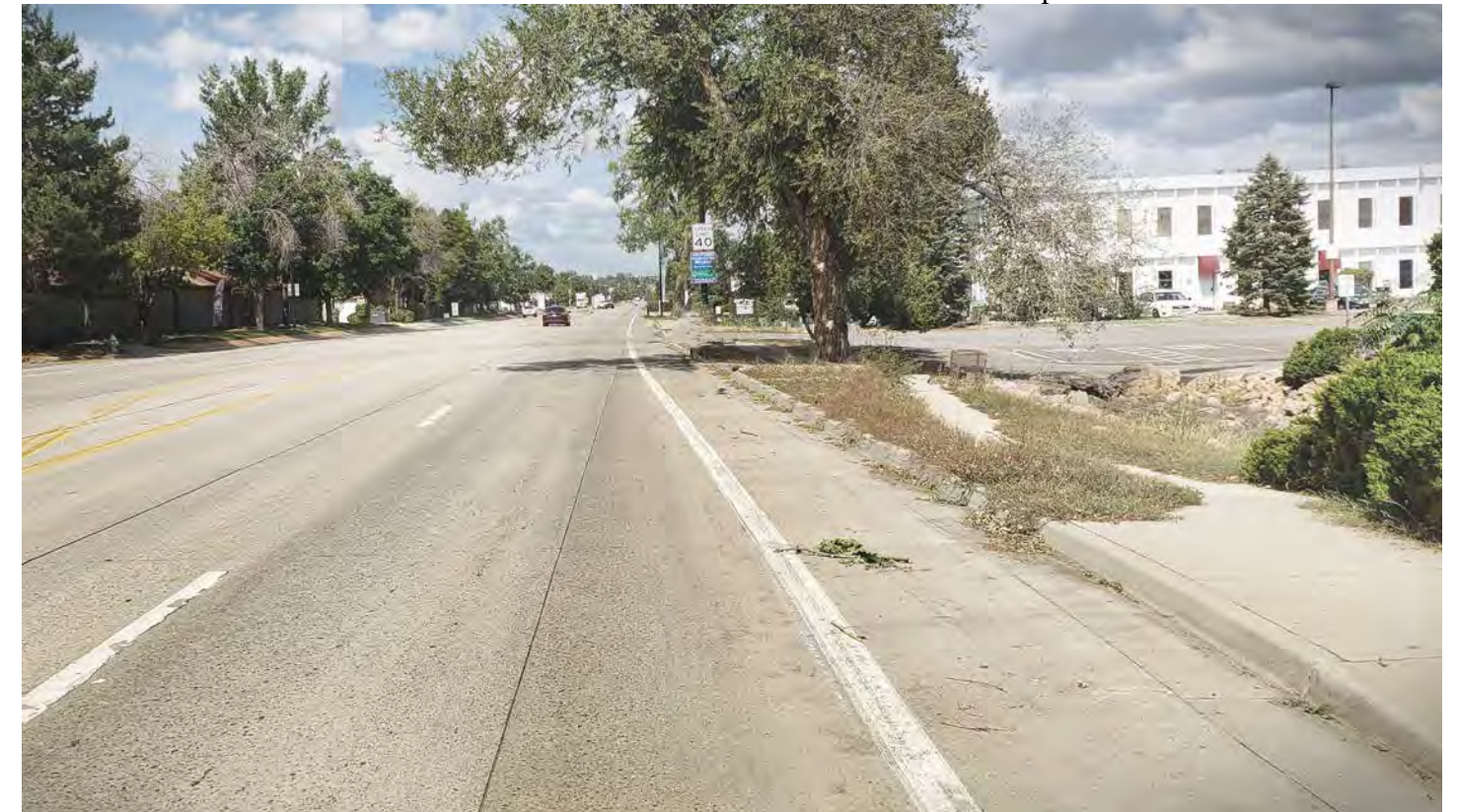
55th Street, Looking North – Existing Condition
