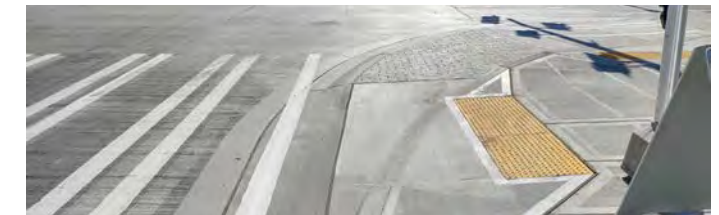
Mountable element, rollover curb example
