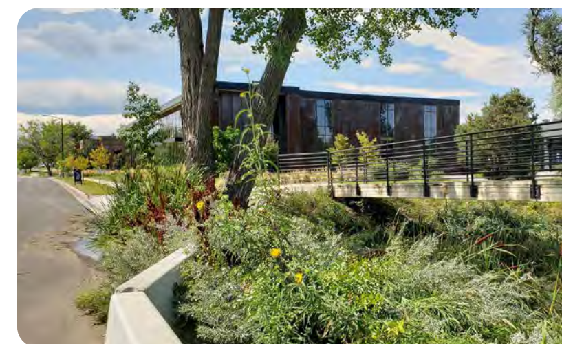
Flatirons Park Stormwater Drainage
