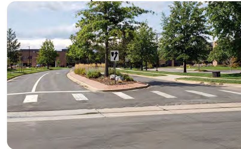
Crosswalk at 55th Street
