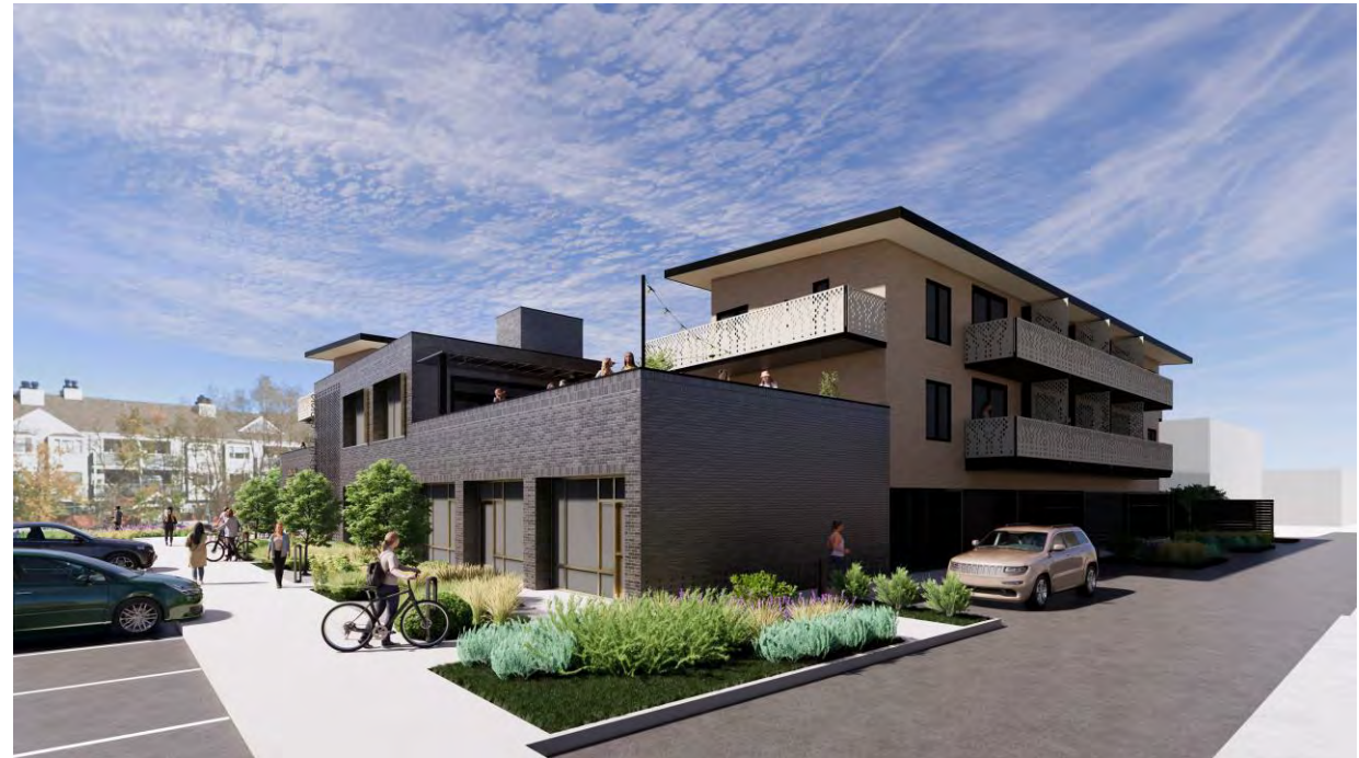
View of southwest corner
