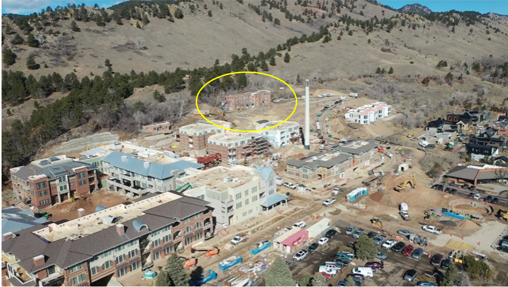
Figure 2. Current site and surroundings. Construction progress aerial footage. 1 Building identifier added by staff.
