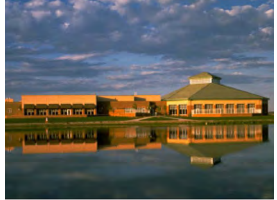
East Boulder Community Center
