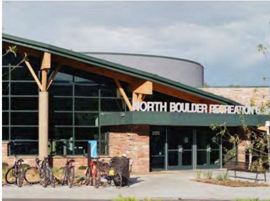
North Boulder Recreation Center
