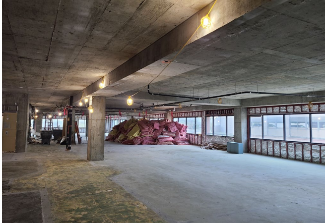
Interior of the Pavilion building, post deconstruction with insulation piled and ready for reuse
