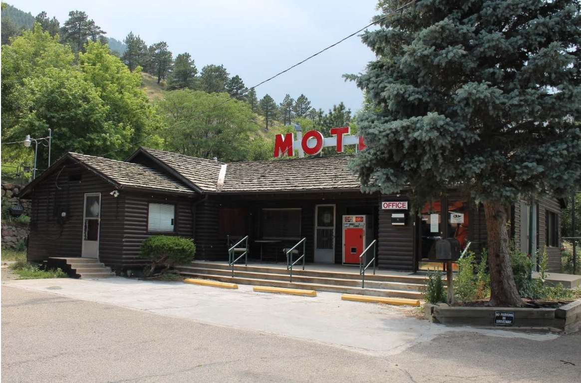
Figure 5. View facing west toward the office administration building, 2018
