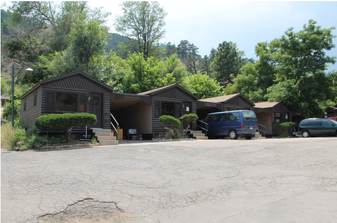
Figure 4. View facing south toward the motel cabins, 2018
