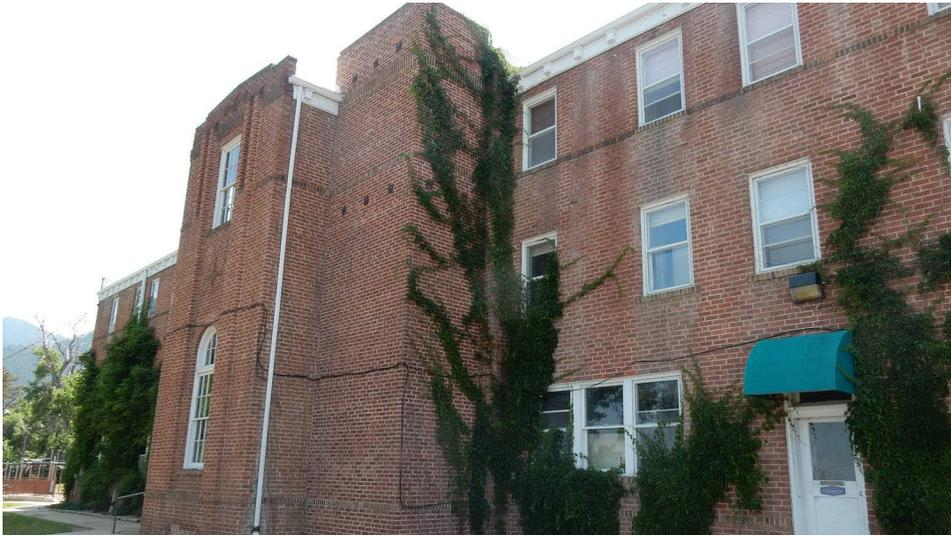
25. The nurse dormitory retains its original brick and architectural features. The only major change is the addition of the elevator shaft which can be seen as the slightly redder brick tower feature.
