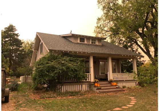
Figure 1. East elevation (façade) of the house from 16<sup>th</sup> Street showing the side gable roof with central shed roof dormer and full width front porch with square porch supports. Provided by applicant.
