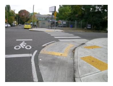
Figure 2-3: Example of A Mountable Truck Apron At An Intersection
